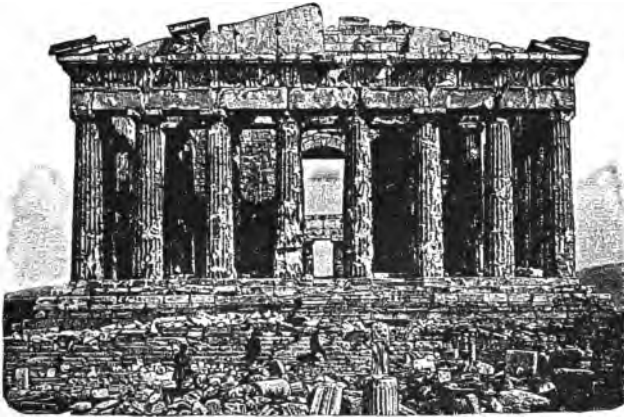
THE PARTHENON (present condition).
